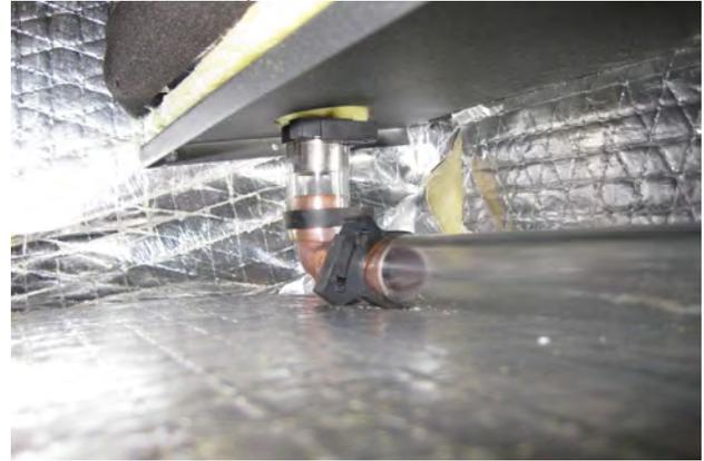
Remove the short piece of vinyl tubing from the drain pan nipple
