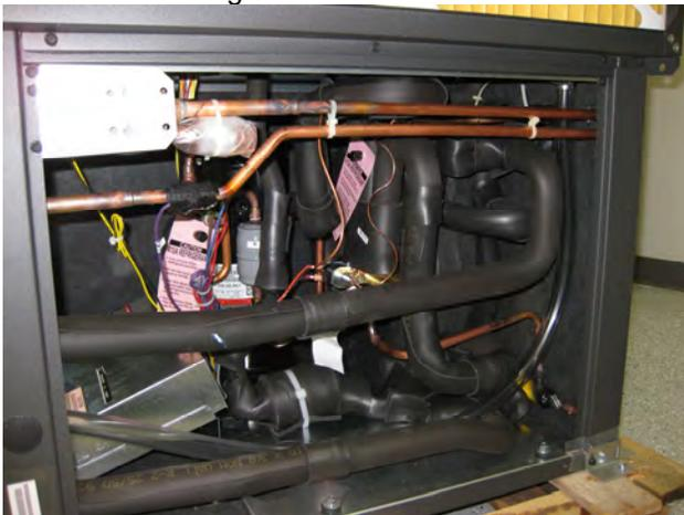
Remove the condensate tubing.
