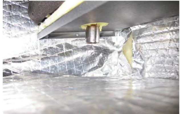
After the condensate tubing is removed, a reciprocating saw with a fine tooth metal blade can be used to cut the “burred” end off of the stainless steel tube. Simply cut approximately ¼ inch off the end. This will remove the burred end and still leave ample length for reconnecting the tubing
