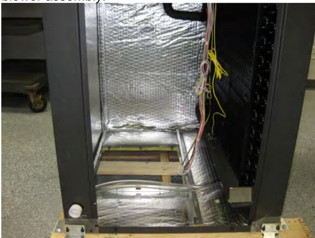
Locate the condensate drain towards the rear of the condensate drain pan
