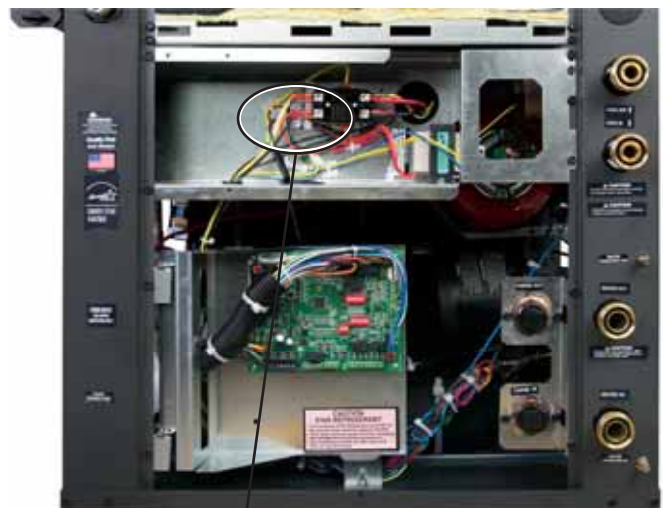
Figure 25: Tranquility Single Phase Line Voltage Field Wiring
