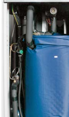
Extended range insulated water/refrigerant circuit standard (shown with optional UltraQuiet mute package)
