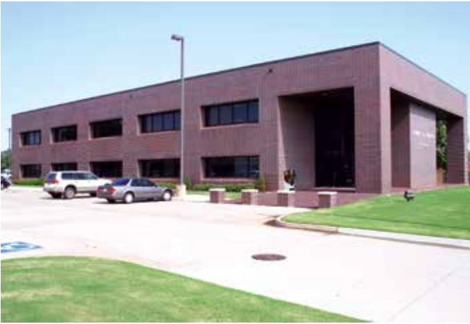
Geothermal loop grid located under the parking area.
