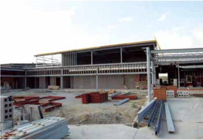
Construction in progress on the school grounds.
