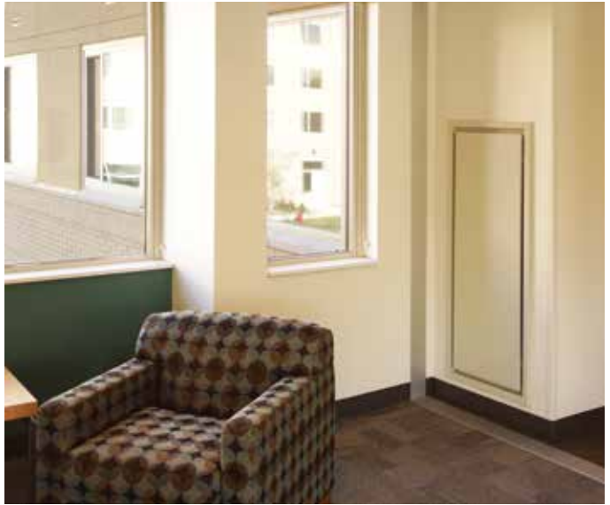
Tranquility Vertical Stack (TRM) units installed in Centennial Hall were finished with attractive return air panels
