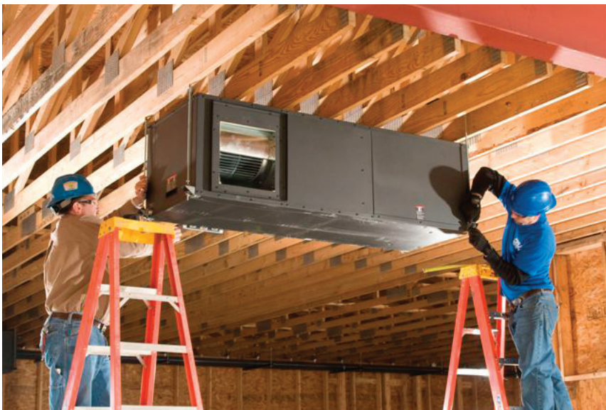
Workers install a ClimateMaster Tranquility geothermal system.
