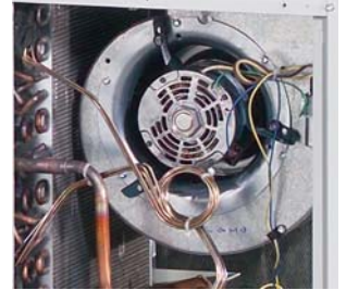
Easy to remove torsion-flex motor mounts for quiet operation and blower inlet ring for quick service (Optional High-Static blowers)
