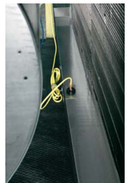
Insulated Drain Pan with condensate overflow protection (Optional Stainless Steel Drain Pan)
