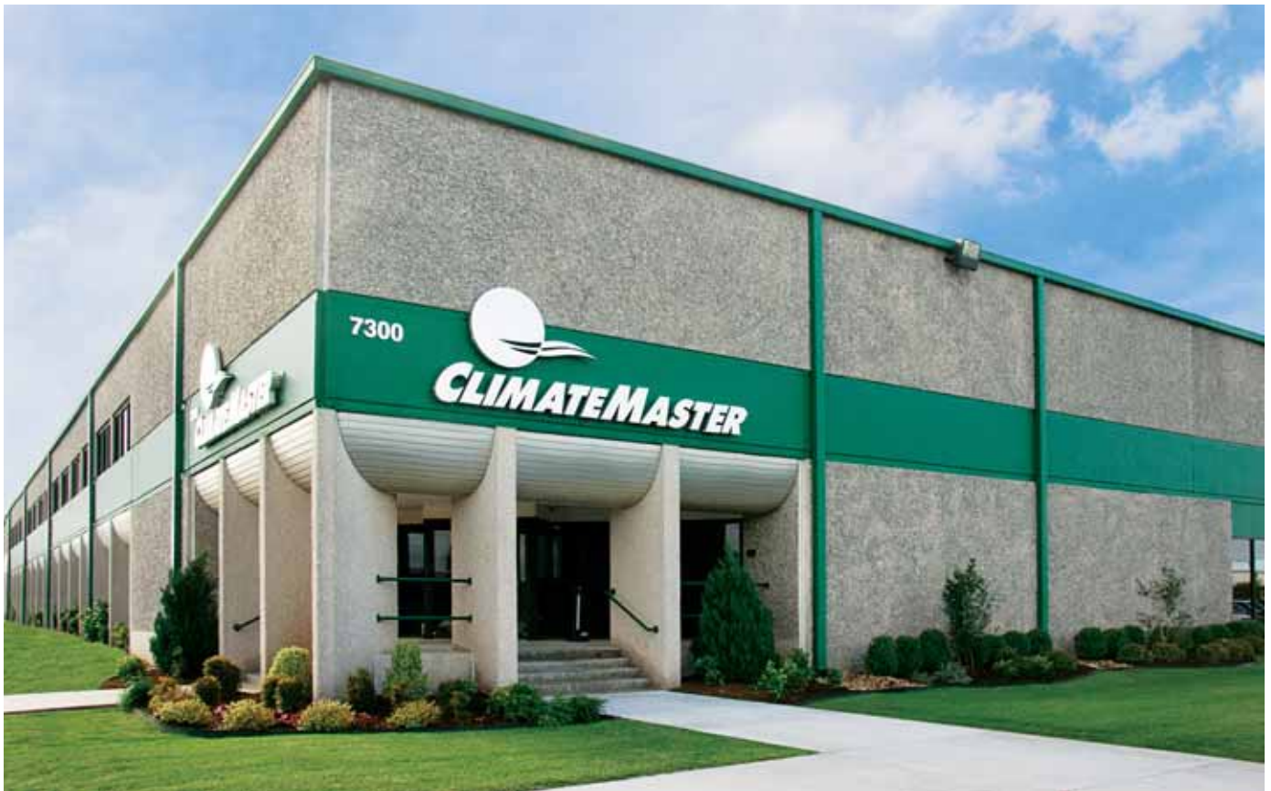
ClimateMaster's manufacturing facility in Oklahoma City, Oklahoma, U.S.A.
